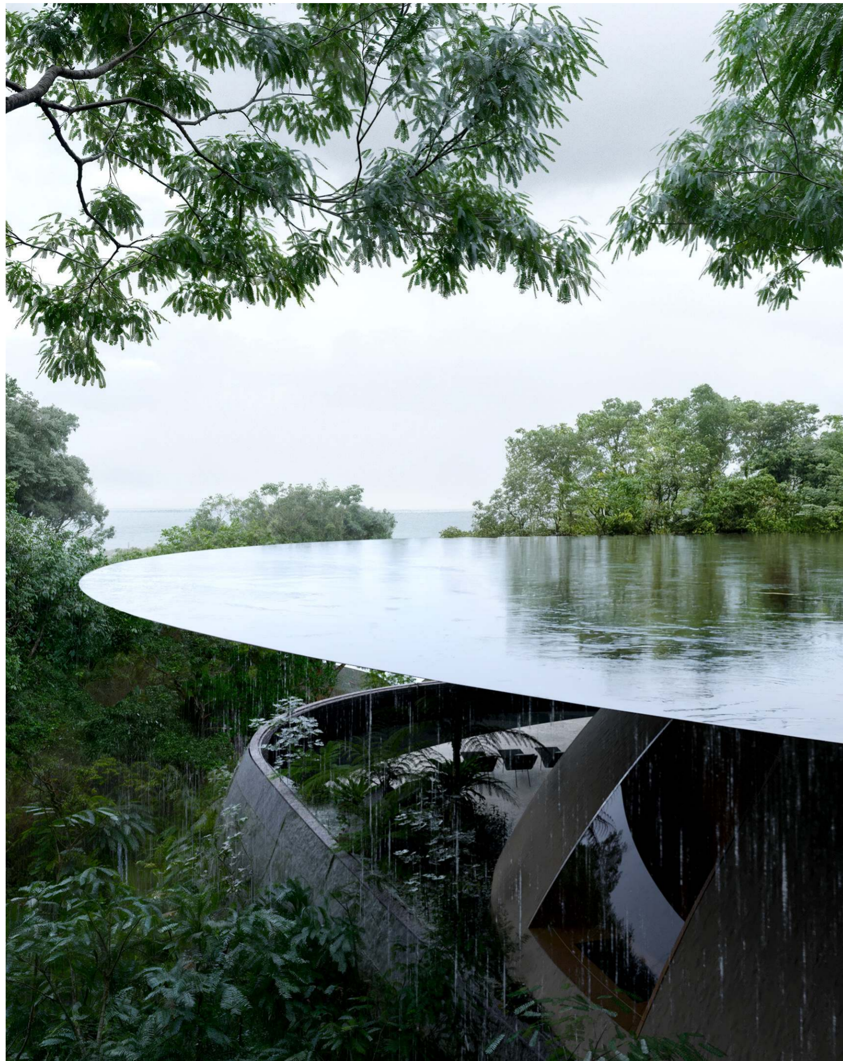
Thin veil of rainwater briefly staged on roof plane before flowing by gravity to filtration, bathing, and water reuse.
